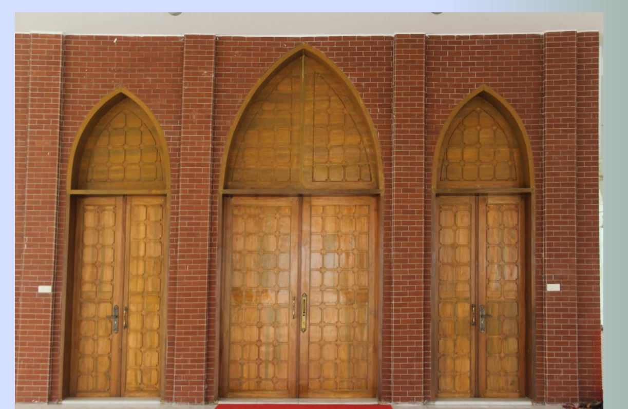
Picture 16 - Wooden Door.
